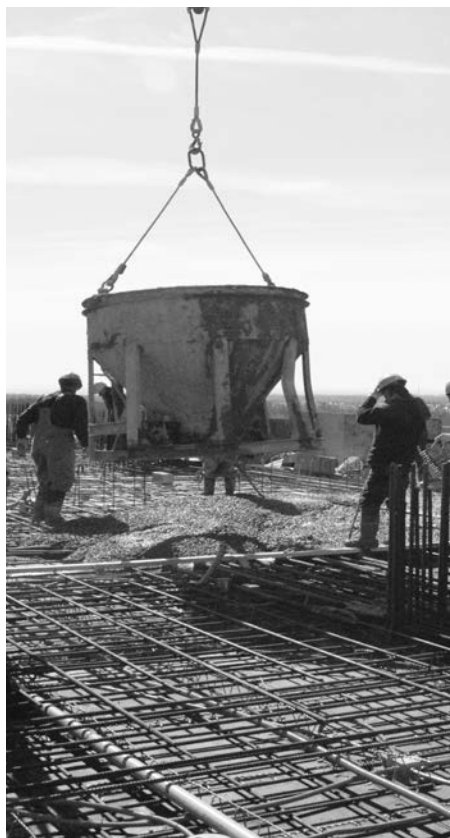
Used to carry fresh concrete from the concrete truck to the point of deposit
