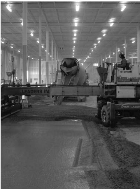
Used to level concrete to a predetermined height
