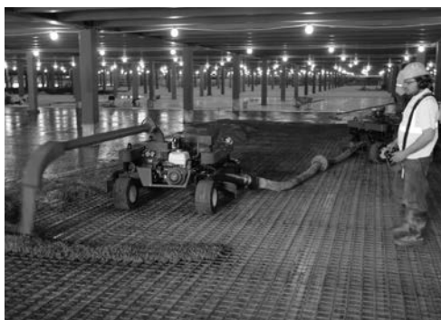
Used to move the concrete pump line mechanically
