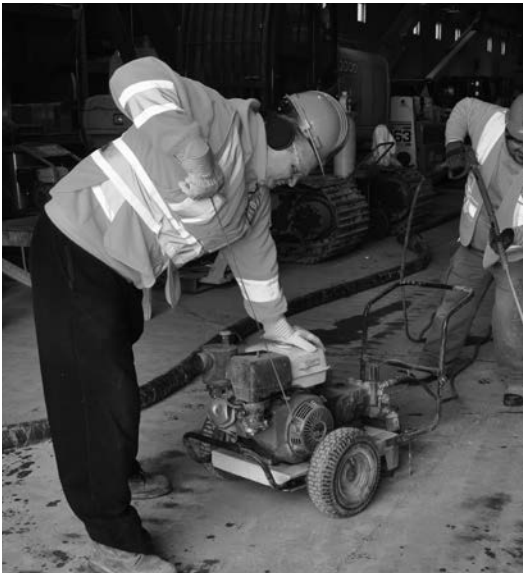
Used to clean concrete before re-sealing
