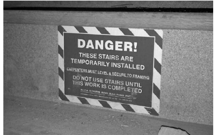
Figure 9-13: Warning sign on temporary stairs
