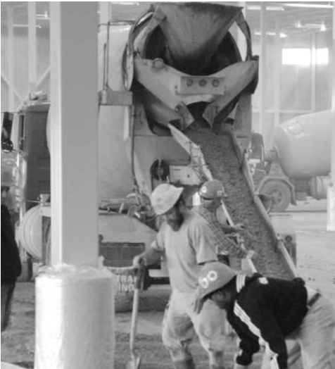
Used to carry fresh concrete from the batch plant to the jobsite
