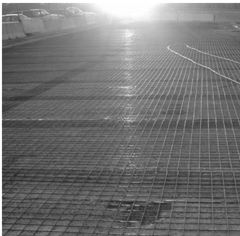
Used to reinforce concrete and create stability across floor joints
