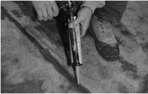
Used to dispense joint sealants and joint filling compounds
