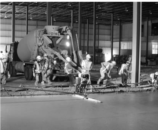
Used to level concrete to a predetermined height
